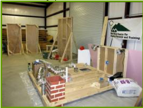
NRCERT training prop for hands-on attic air sealing and insulation prep
