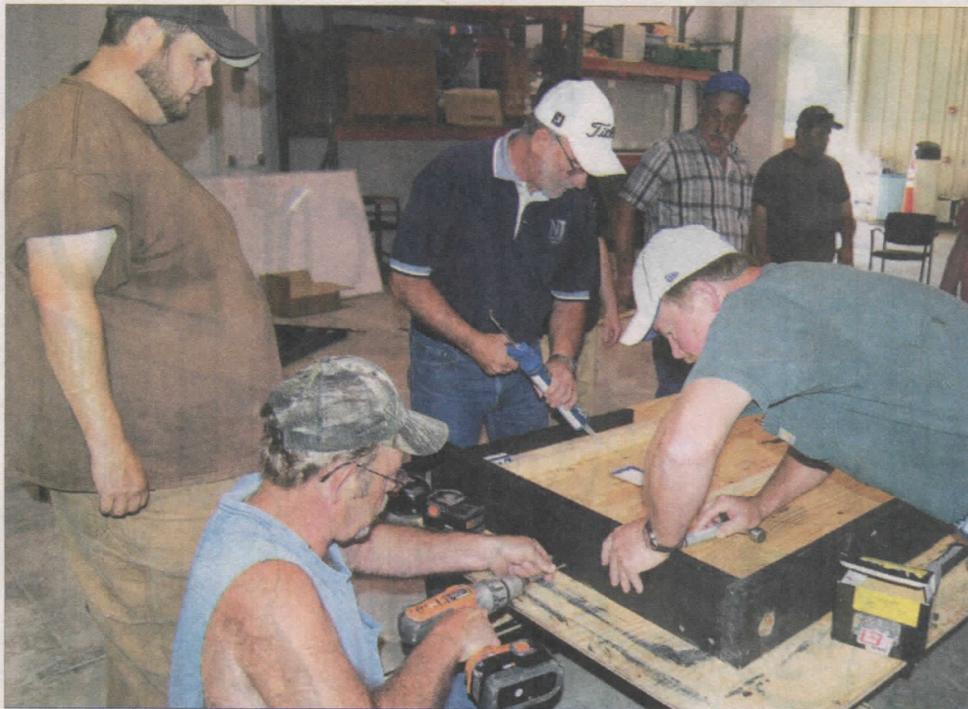
Building trades workers in the solar installer class at Wytheville Community College's campus at the Crossroads Institute in Galax pitch in on several tasks all at once while building a solar powered water heating system. The students will make the system operational and see how effective it is.
