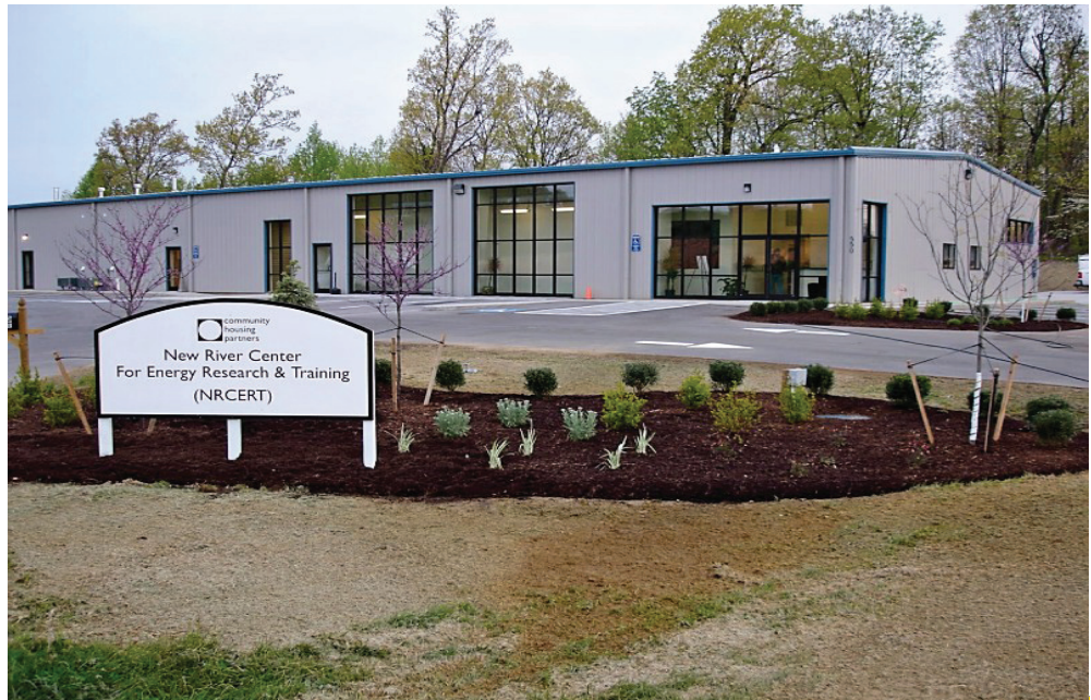
The NRCERT Weatherization Training Center completed its expansion in March 2010 and provides over 12,500 square feet of hands-on training area.
