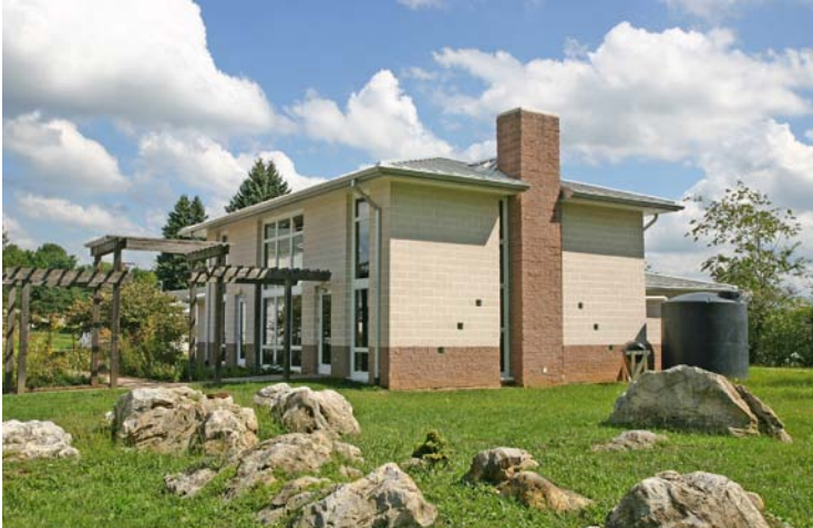
FIGURE 6. Dining Hall exterior with rain cistern.
