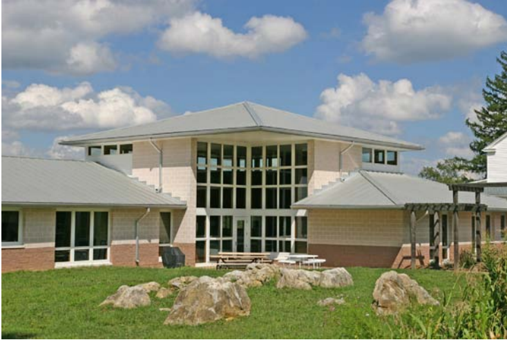
FIGURE 12. Rear exterior view of Dorm-Administration building and outdoor courtyard.
